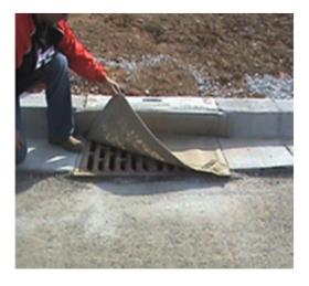
3. Catch Basin Filter Cover with overflow protection with insert in basin
