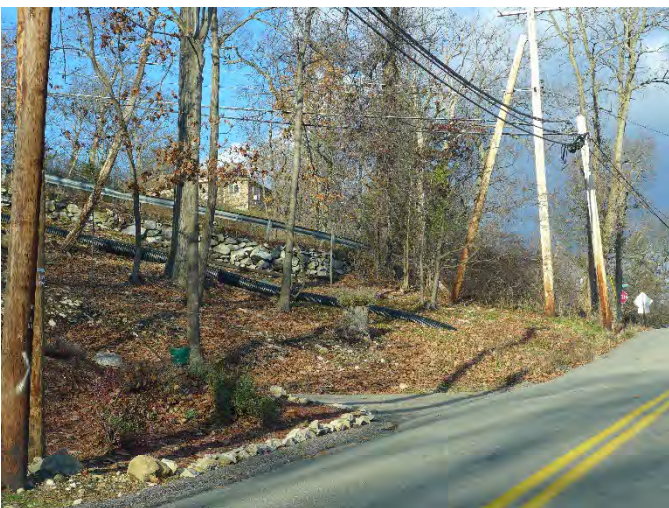
Photo 10: Tanglewylde Road existing overland piped conveyance potential for conversion to stabilized vegetated conveyance system.
