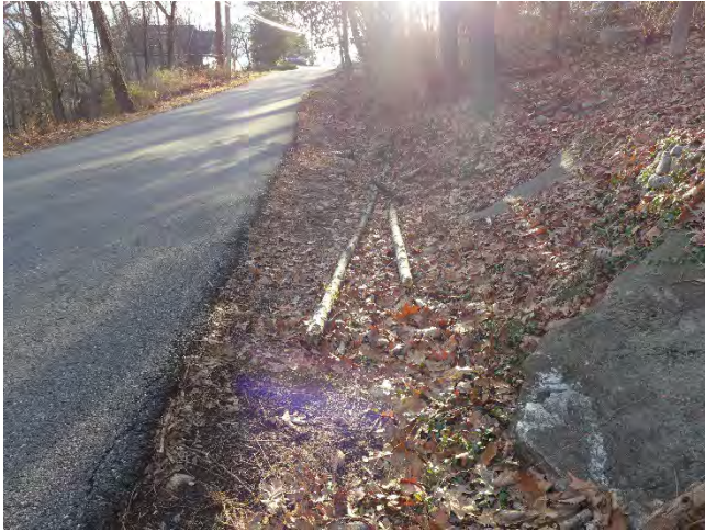
Photo 23: Pleasant Road existing ditch and culvert pipe; looking south.
