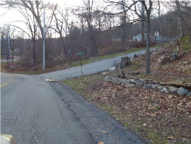
Photo 9: Tanglewylde Road existing asphalt ditch with potential for conversion to bioswale prior to entering drain.
