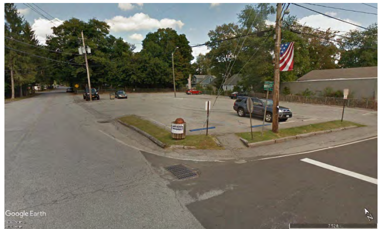
Photo 32: Outlet of parking lot drainage
