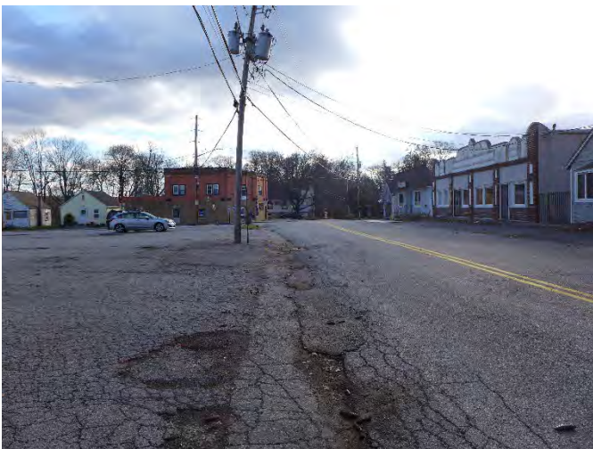
Photo 31: Parking Lot, Looking south
