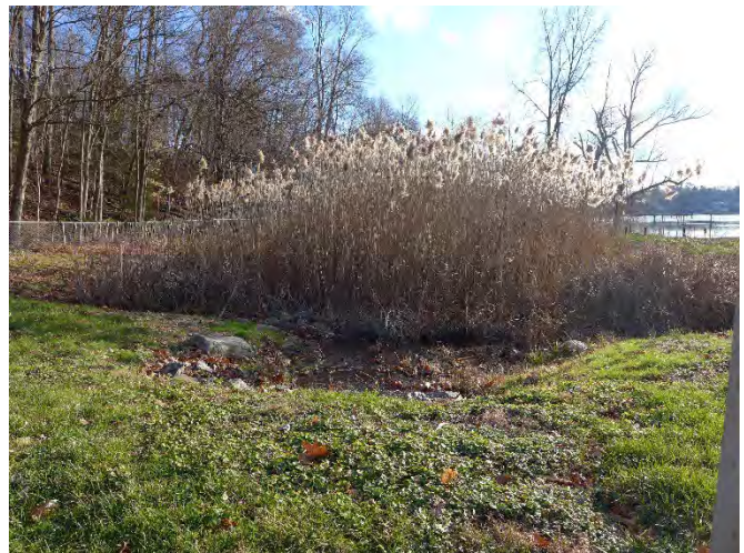
Photo 65: Entry of piped flow to existing wet basin.
