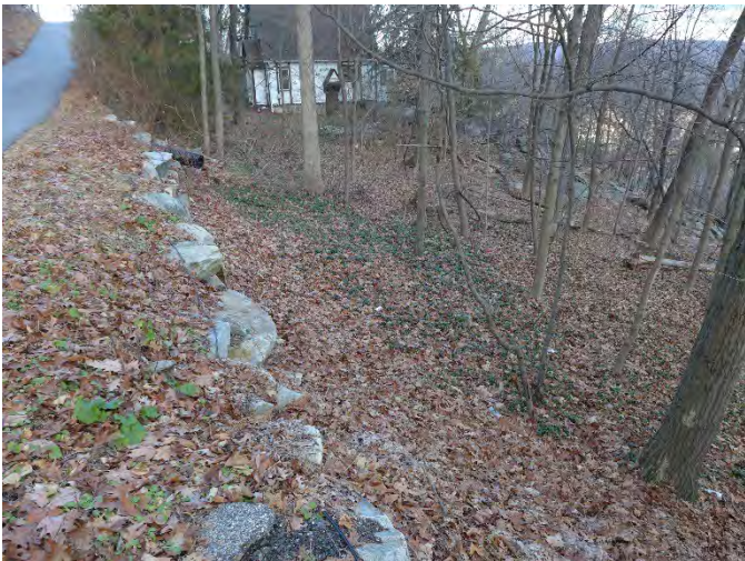
Photo 11: Site 6A Culvert discharge point draining to steeply sloped wooded area.
