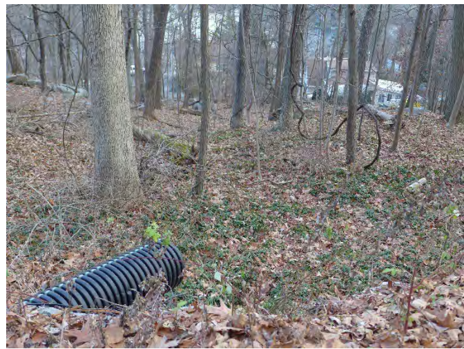
Photo 12: Site 6A Discharge Location of 12 in. HDPE pipe
