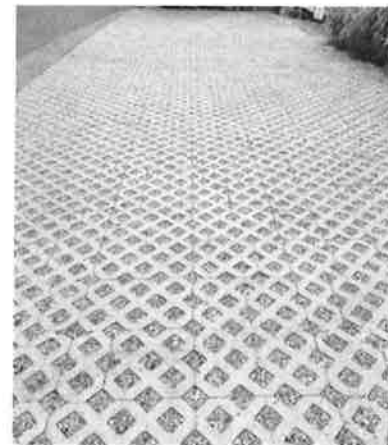
Photo 4 Oscawana watershed interlocking pavers filled with pea-gravel
