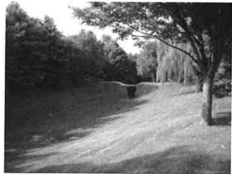
Photo 1 Dry Detention Basin ( https://sustainablestormwater.org )
