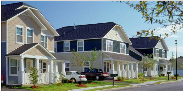
A row of duplexes that have been designed to be indistinguishable from single-family detached homes
